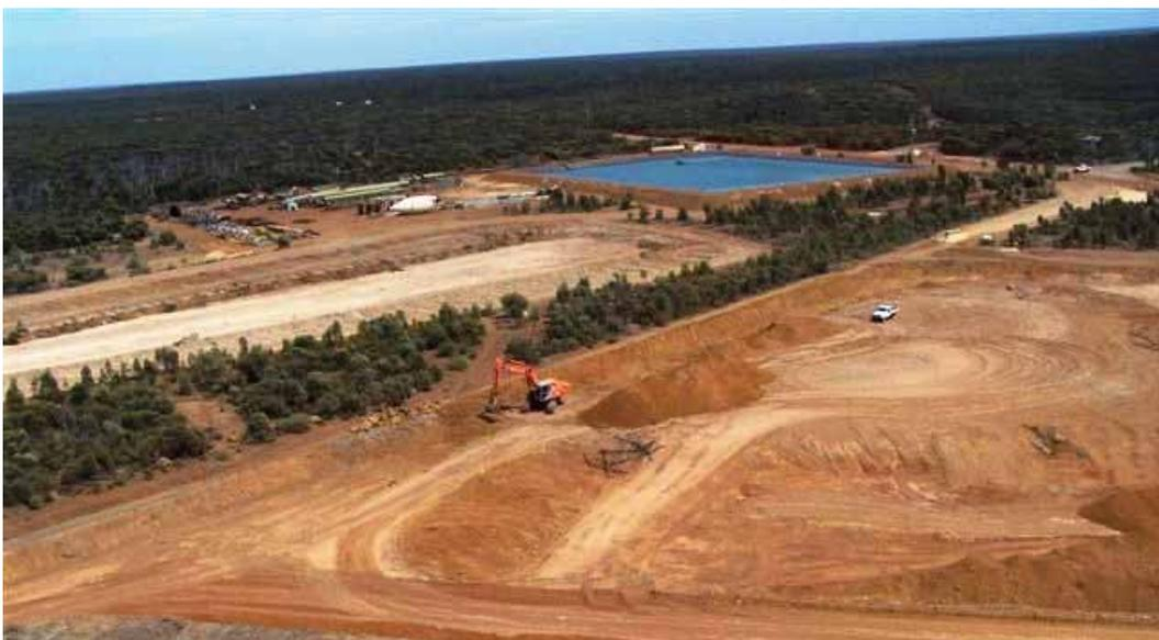
**Figure 2:** Cosmic Boy concentrate plant site showing water storage and Cosmic Boy mine boxcut which is being excavated to provide fill for the plant ROM pad and access to remnant ore in the mine.
