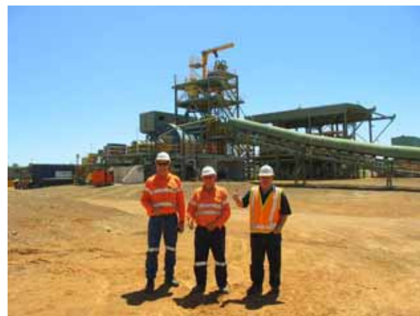
Coarse ore bin on LHS background, concentrate shed and filter on LHS foreground, workshop/store on RHS foreground, the SAG mill, flotation plant and thickener in centre and ROM pad and crusher in background.
