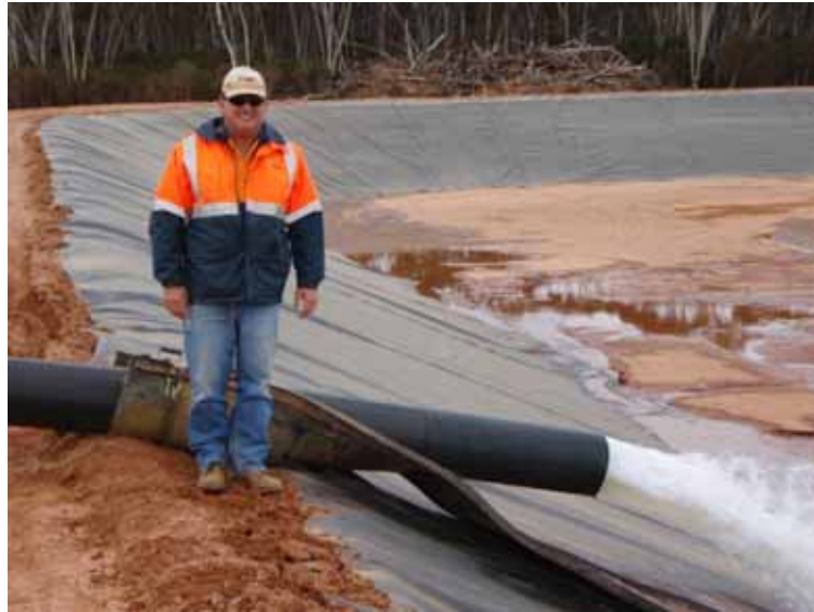
Figure 5: Water from Digger Rocks mine flowing into the newly completed evaporation pond
