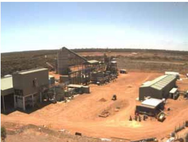
Coarse ore bin on LHS background, concentrate shed and filter on LHS foreground, workshop/store on RHS foreground, the SAG mill, flotation plant and thickener in centre and ROM pad and crusher in background.
