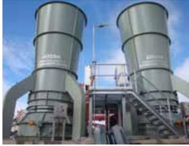
Figure 2: Primary mine ventilation fans installed at Flying Fox
