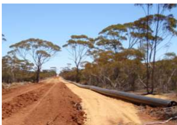
Installing dewatering pipeline from Diggers South to Mossco Farm
